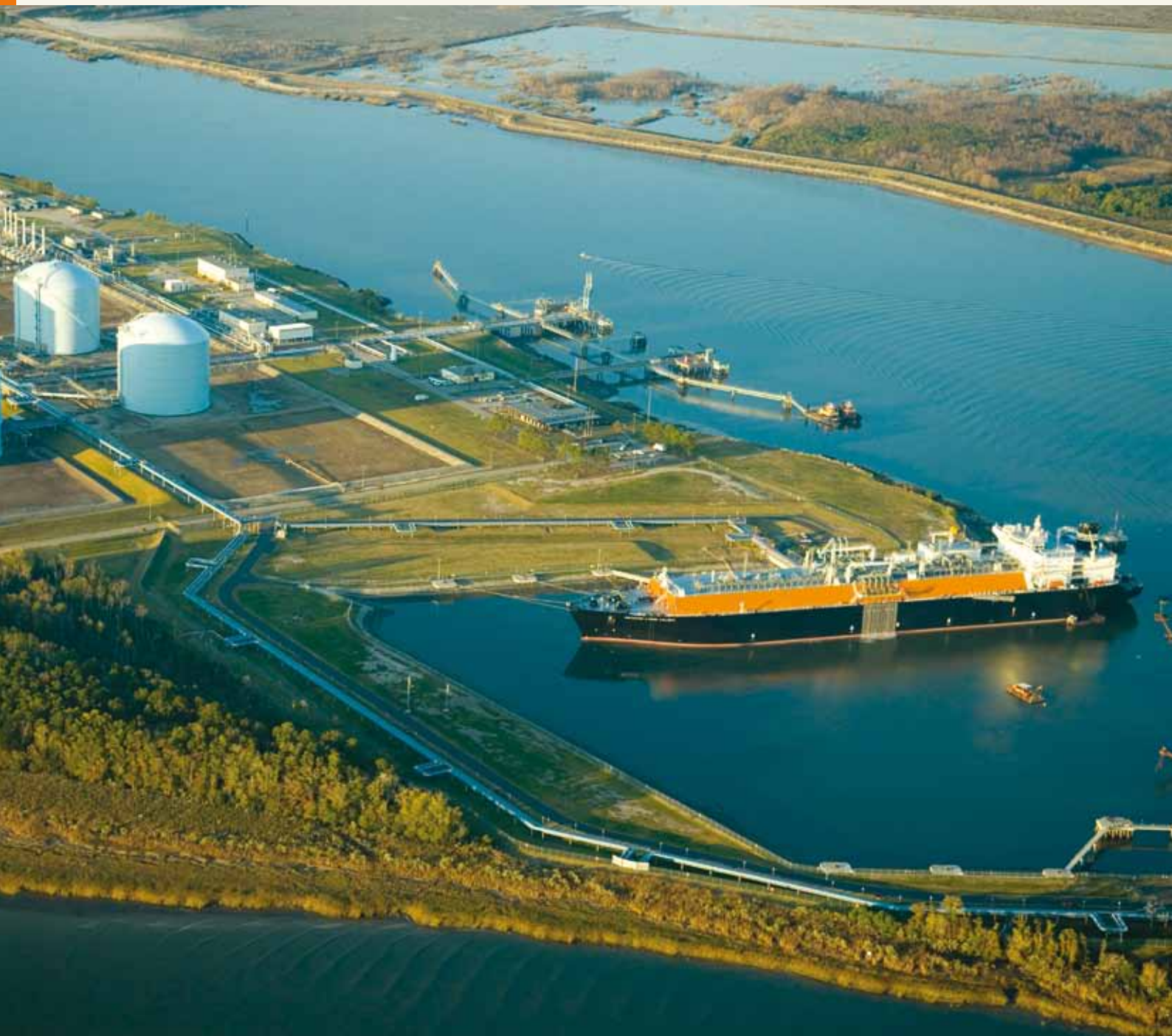
Elba Island regasification plant in Georgia, United States
